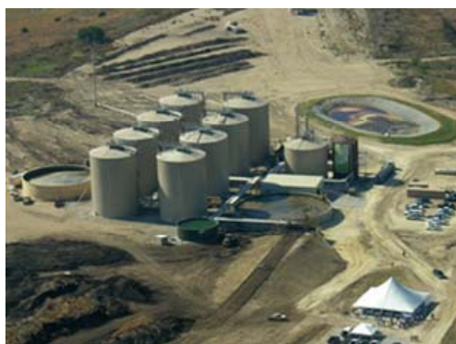
Figure 10: Microgy Inc biogas production and conditioning facility in Texas. source: Microgy Inc.
